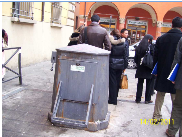
Under Ground Waste Disposal
